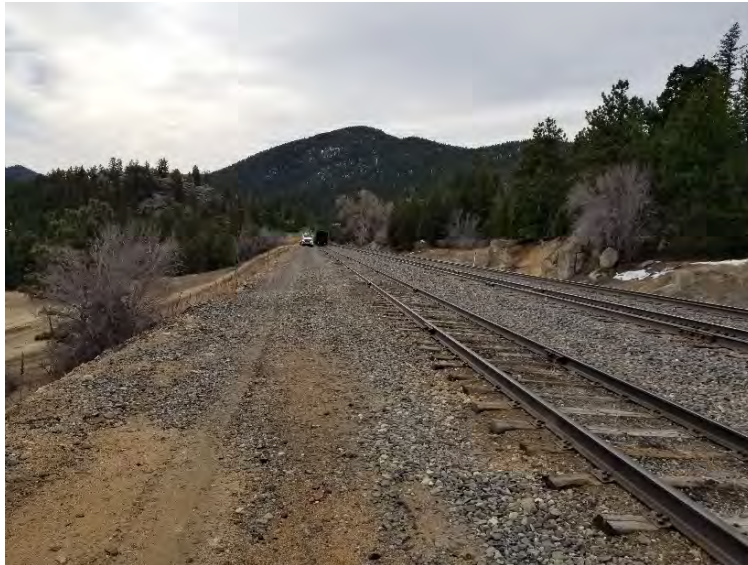
UPRR Crescent Siding, Trucks Parked Near Unloading Area from Left to Right, Siding Track, Parking Track and UPRR Main Line
