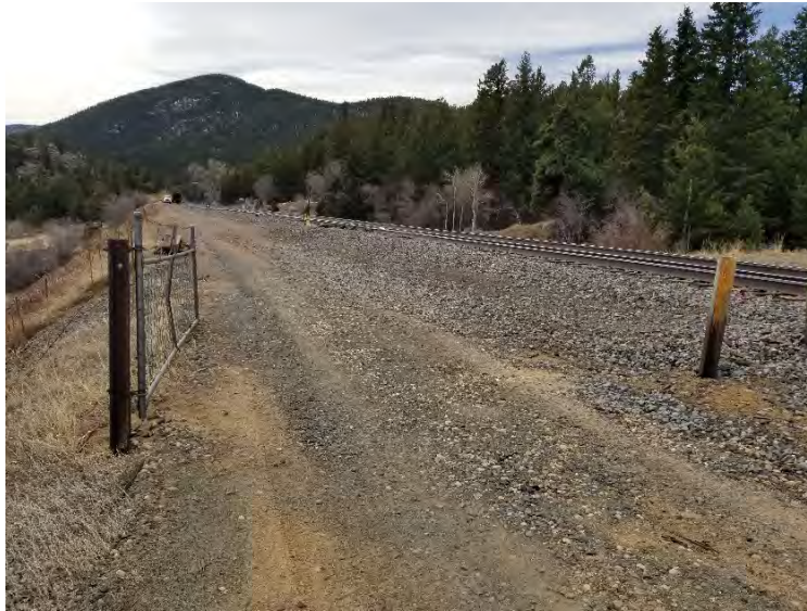
UPRR Access Road Crescent Siding
