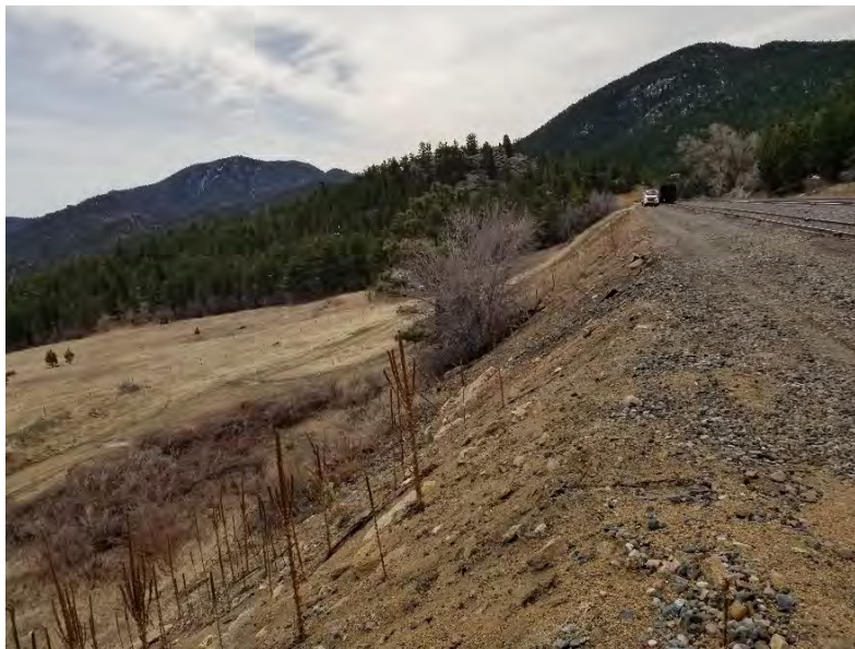
Future Terminal and Silo Area
