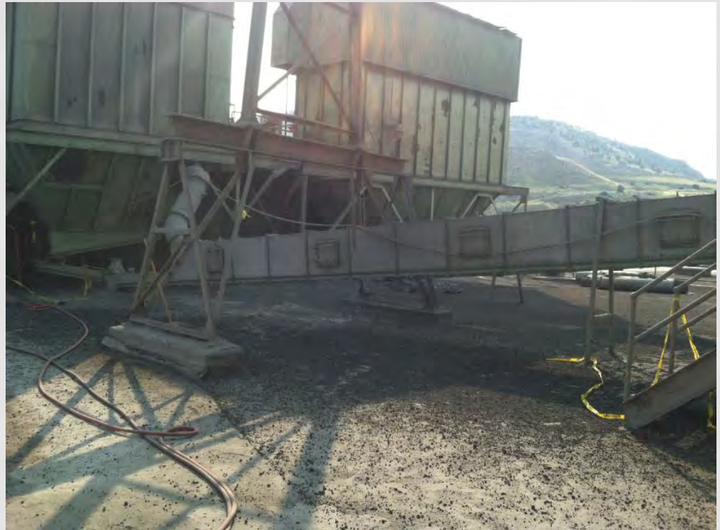
Holcim Trident Site - Crescent Siding Facilities (from D Hertel email 7/21/14)
