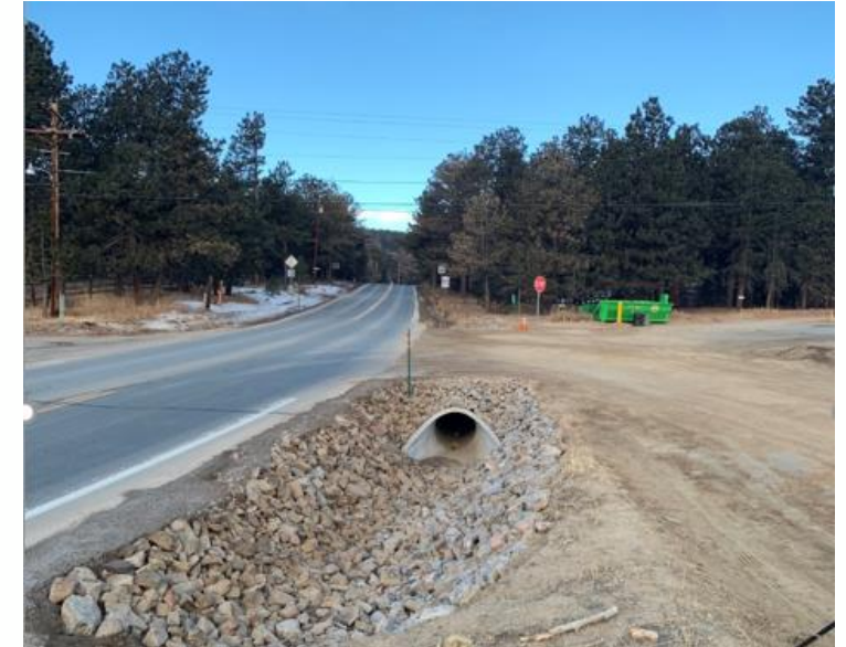
New Culvert at Gross Dam Road
