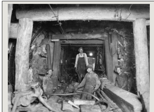
Workers pose for a photo in the Moffat Tunnel in this 1930 photo.
