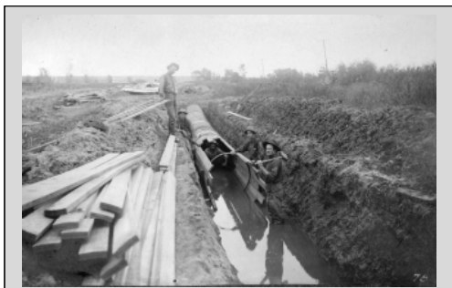
Workers build a wood-stave pipe in this undated photo. In the early 1900s, many of Denver Water's conduits and large pipes were made of wood.
