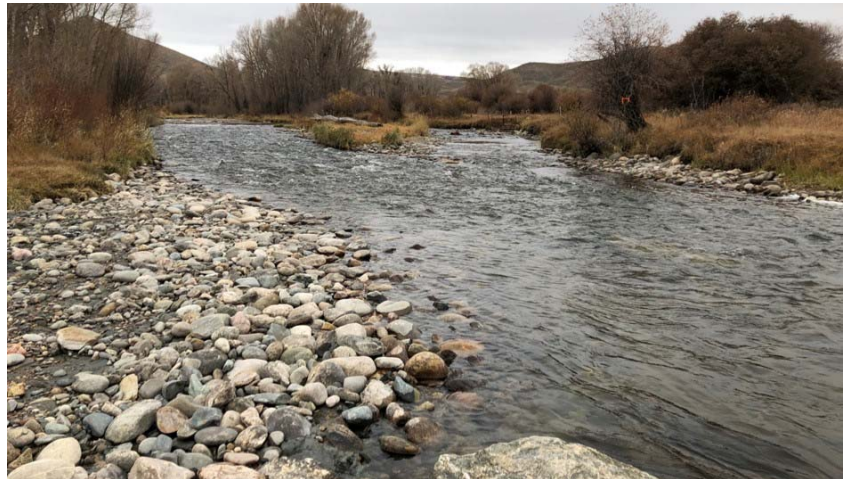
Williams Fork restoration work
