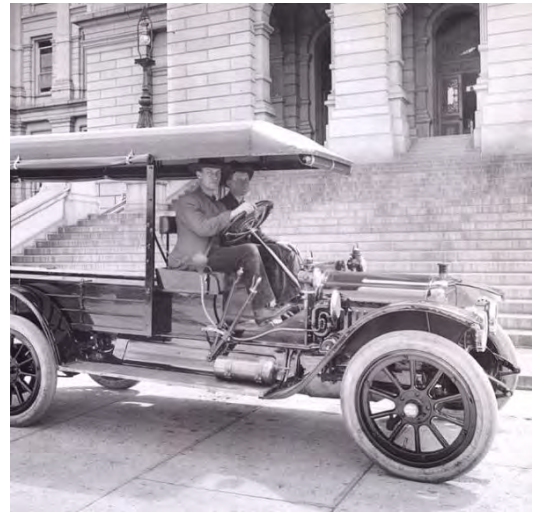
A hydrant repair motor truck making it's rounds at the State Capitol, June 1913
