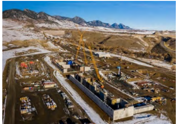
Northwater Treatment Plant under construction, October 2020
