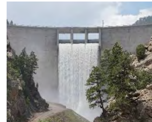
Strontia Springs Dam Spillway, 2019
