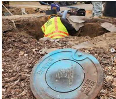
Pieces of lead service lines installed by builders decades ago. Denver Water is replacing lead service lines with new, lead-free copper lines at no direct charge to the customer.
