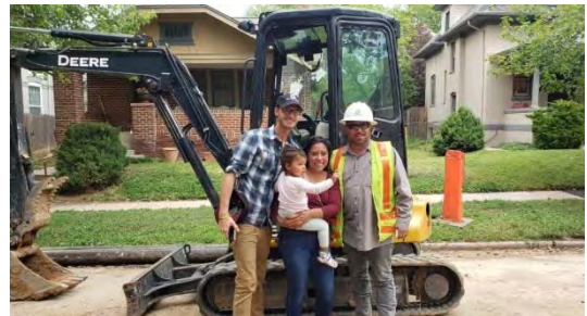
Customers stop by worksite to meet Denver Water equipment operators, 2020.
