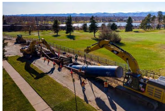
Construction crews install a 50-foot section of steel pipe next to Willis Case Golf Course in northwest Denver. Large pipes are 66 inches in diameter and weigh 11,500 pounds, 2020.
