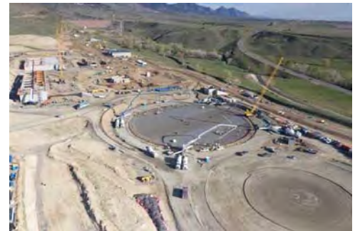
Northwater Treatment Plant being built between Ralston Reservoir and Highway 93.
