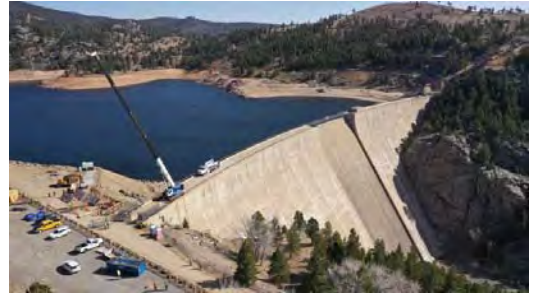
Gross Dam Expansion, April 2022.
