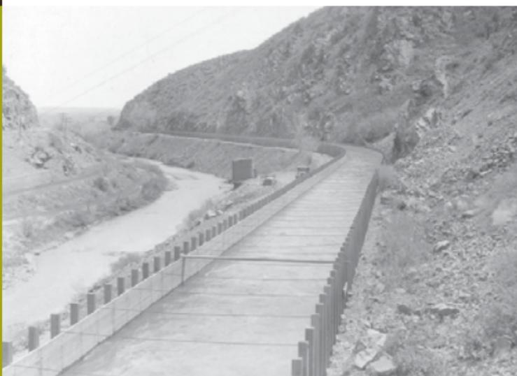
*This 1935 photo shows the High Line Canal carrying 275 cubic feet of water per second.*
