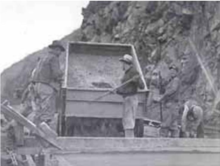
*Crews place concrete in the floor slab of the High Line Canal Canyon Flume in this 1934 photo.*
