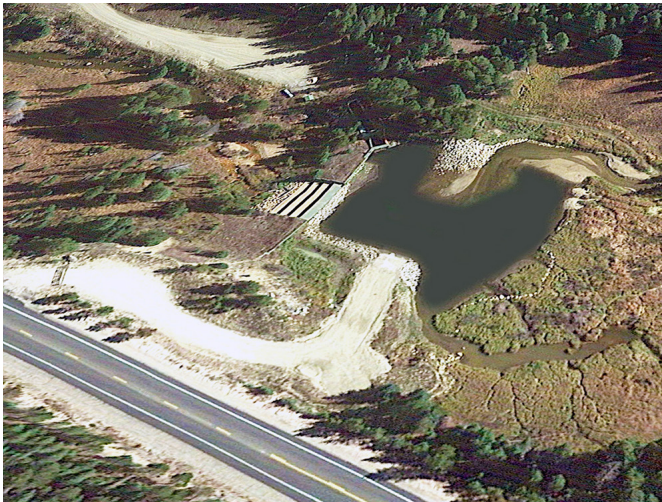
Denver Water reconfigured the pond for traction sand collection and removal. Photo credit: Google Earth.
