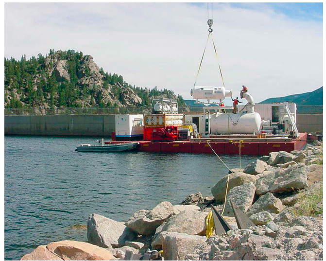
Progress of the Outlet Works Modification Project. Photo credit: Denver Water.
