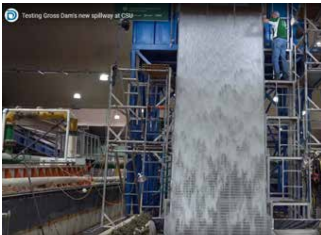
The Gross Dam spillway directs overflow water through the center of the dam. Photo credit: Denver Water.
