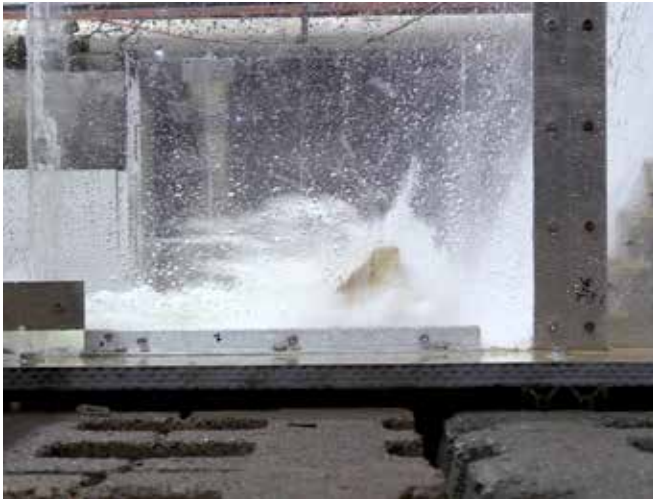
The stilling basin, shown above, is located at the bottom of the dam and slows water that flows down the spillway. Photo credit: Denver Water.
