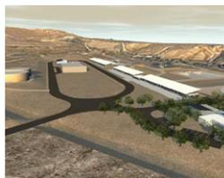
**Northwater Treatment Plant:** We are building a new, state-of-the-art water treatment plant next to Ralston Reservoir, north of Golden in Jefferson County. The Northwater Treatment Plant will be capable of treating up to 75 million gallons of water a day and will be equipped with disinfection technology that will provide more flexibility to react to changes in water quality.
