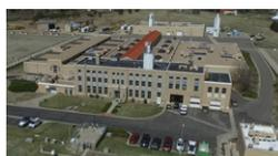
**Moffat Facility:** This facility will continue to treat water although at a reduced capacity. Water treated at the Northwater Treatment Plant will be sent to the Moffat Facility, via the Northwater Pipeline, where it will be stored and distributed to customers.
