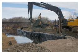
**Northwater Pipeline:** We are installing a 66-inch diameter pipeline, replacing one of the two existing pipelines, running 8.5 miles between Ralston Reservoir and the Moffat Treatment Plant. The new pipeline will transport treated water from the new Northwater Treatment Plant to the Moffat Facility for distribution.
